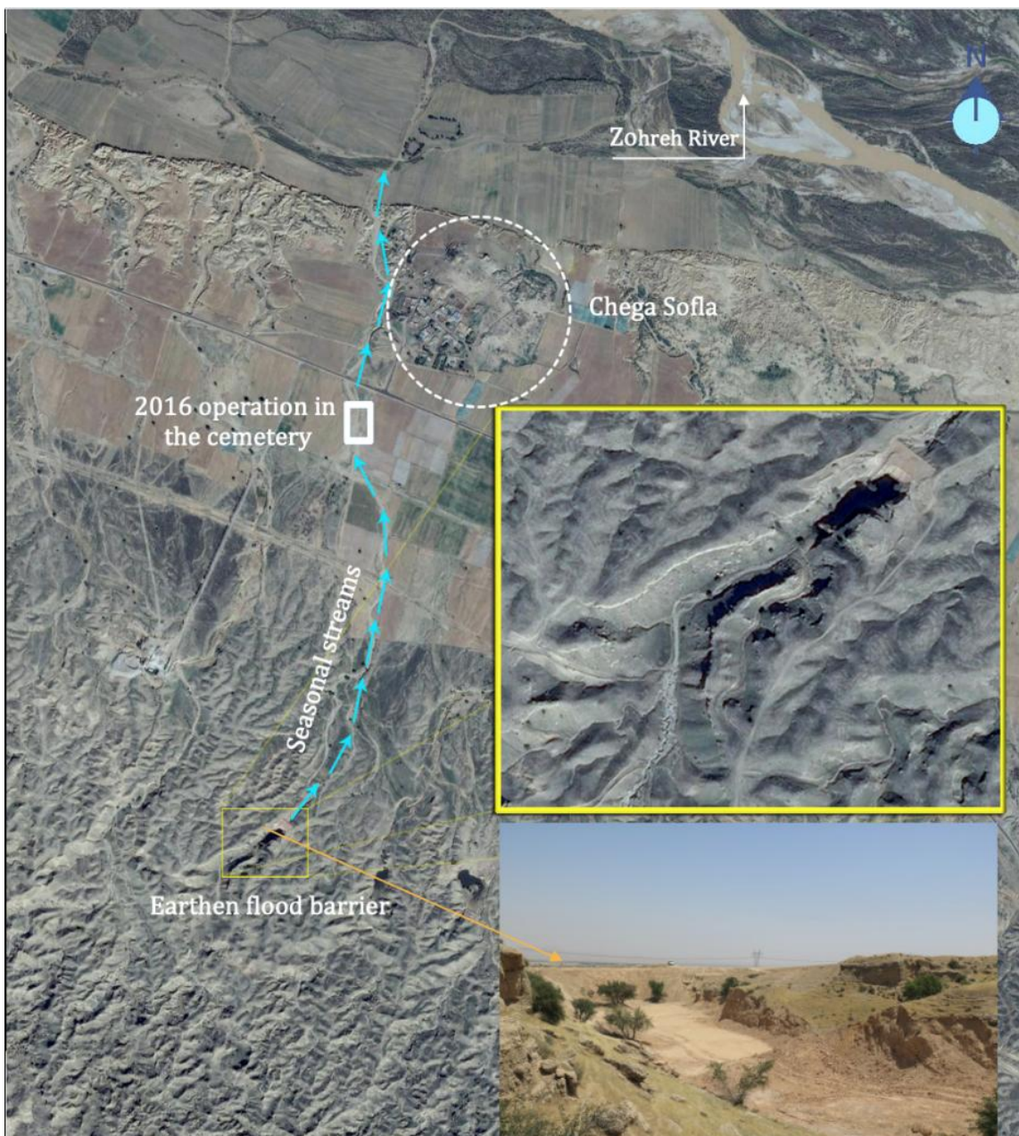
Figure 10. Creating an earthen dam to protect the cemetery and the western wall of the Chega Sofla compound.
