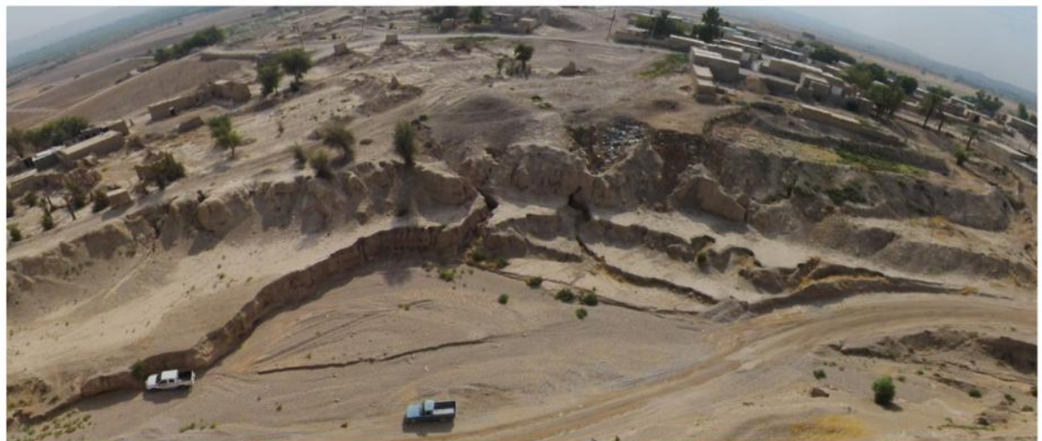
Figure 9. The western wall of Chega Sofla and extensive erosion due to the activity of the western gully of the site over the past years (aerial photo by Loghman Ahmadzadeh).
