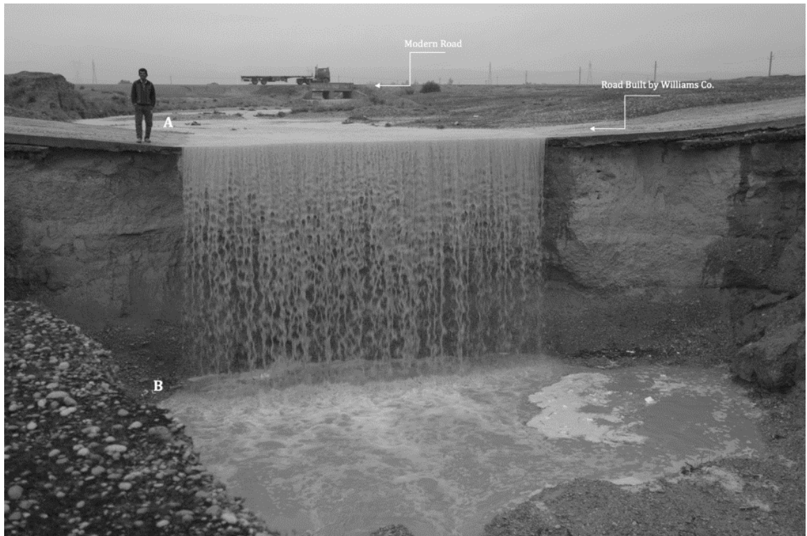
Figure 4. The image, captured during the heavy rains of February 2017, clearly illustrates the long-term impact of the Williams Company's substandard road construction on the plain's natural drainage system. The elevation difference between points A and B highlights how the poorly built road has disrupted the landscape over several decades.
